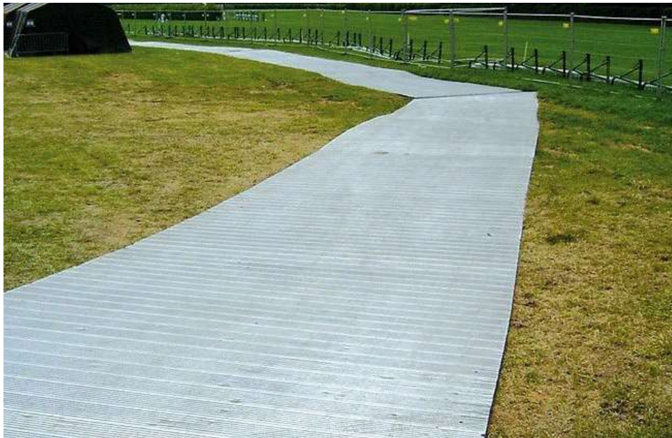
Figure 3-8: Temporary Aluminium Access Trackway
